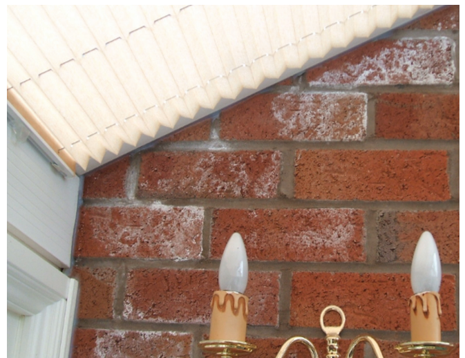
Figure 28: - Masonry walls - acting as a retaining wall
